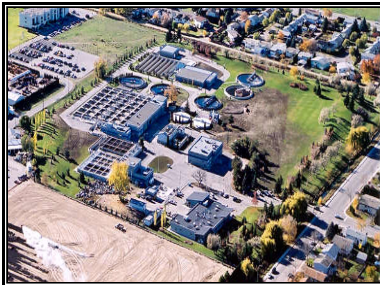
Kelowna’s Wastewater Treatment Facility (WWTF)
