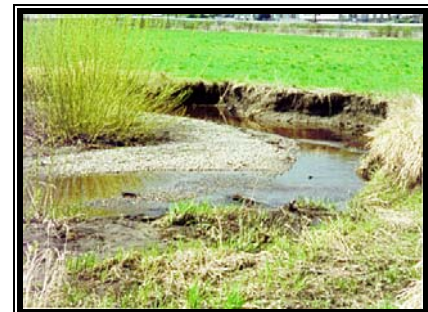
Mill Creek – Streambank erosion
