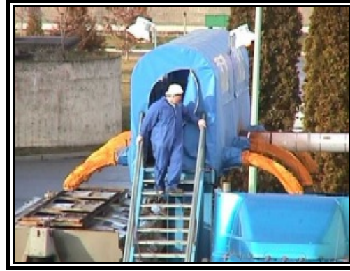
Kelowna’s Wastewater Treatment Facility (WWTF)
